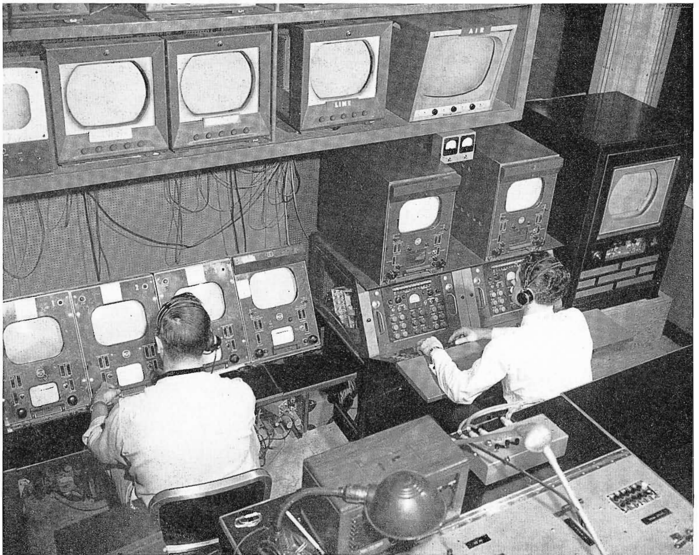
FIG. 18. Lower level of studio control room, showing video control equipment. At left, monochrome; at right, color.
