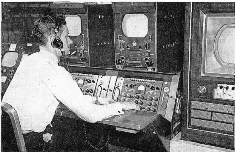
FIG. 12. Operating position in studio control room for two color cameras.
