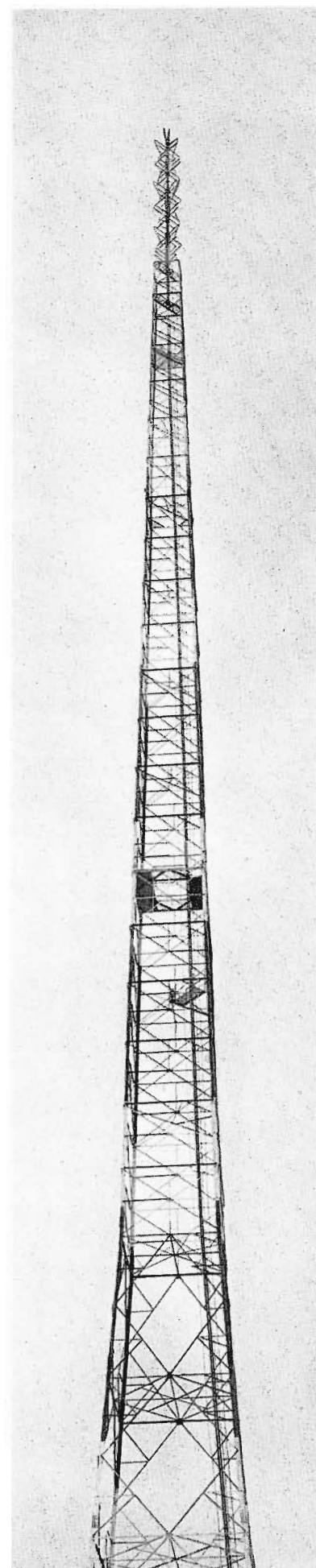
FIG. 27. Station uses an RCA 6-bay superturnstile that radiates an effective power of 100,000 watts.
